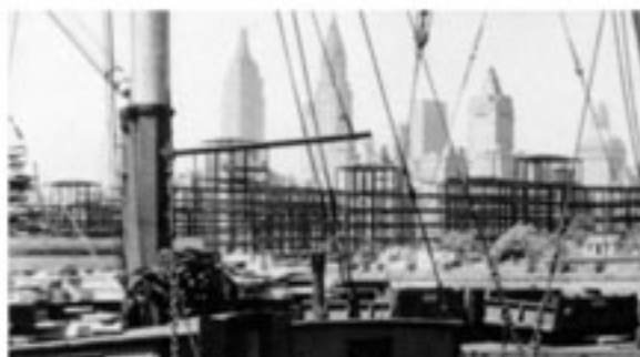
Goldwater Hospital under construction, 1937
