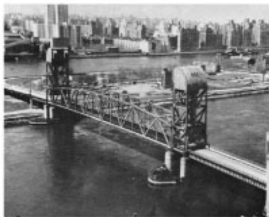
Above, Welfare Island Bridge, ca. 1969. Right, Roosevelt Island Bridge, 1999.
