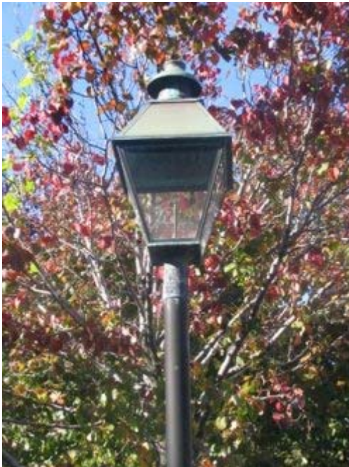
The street gas lamp was unlit.
