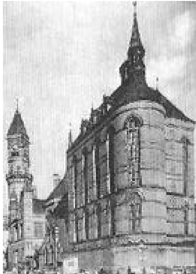
Jefferson Market jail. Behind it the court & tower.
