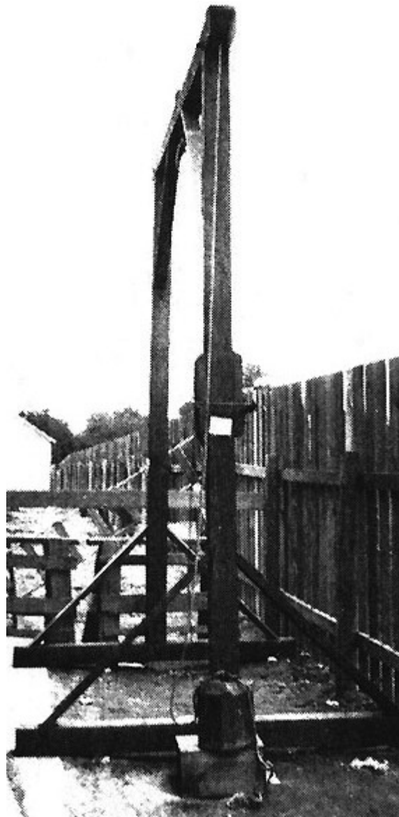
A gibbet -- perhaps similar to the example shown above from Genesee County, N.Y. -- apparently was employed in hanging executions at Brooklyn's Raymond Street Jail and NYC's Tombs. Such a device was operated by using a counter weight, which when released, caused the rope to pull the noosed condemned criminal up with such sudden force as to break the neck (if done correctly).
